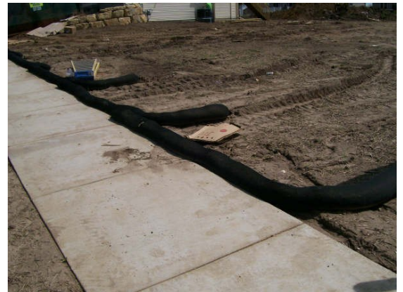
Curl sock ends out in heavy flow areas.
